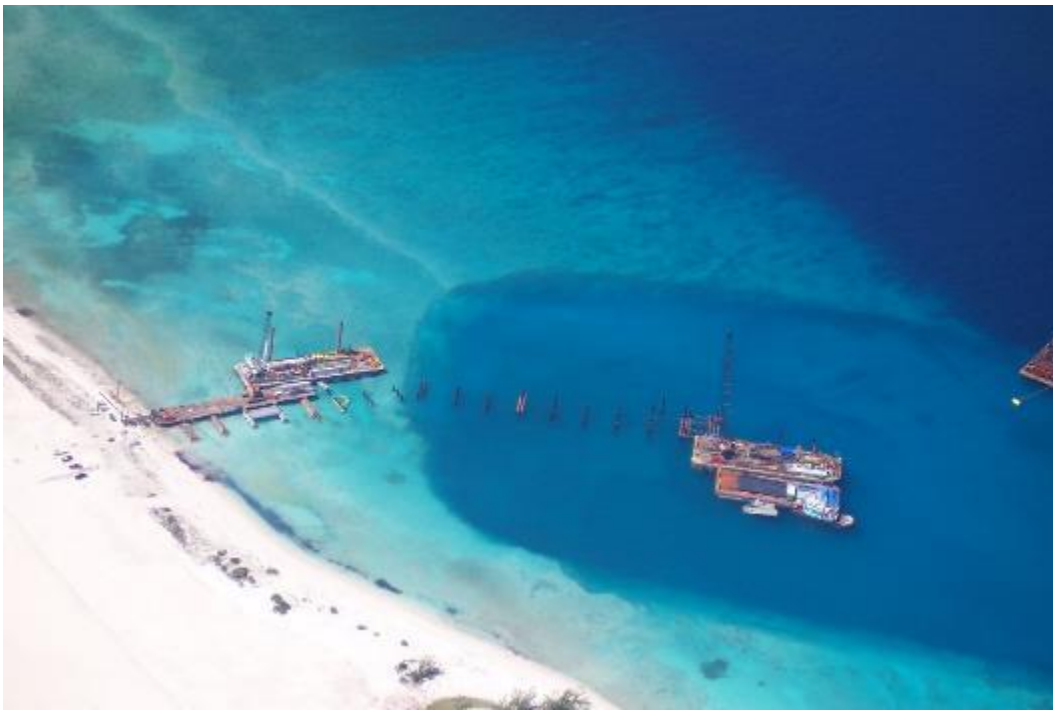
Photo 6.3. Representative photo of pile driving (Grand Turk Cruise Facility construction)
