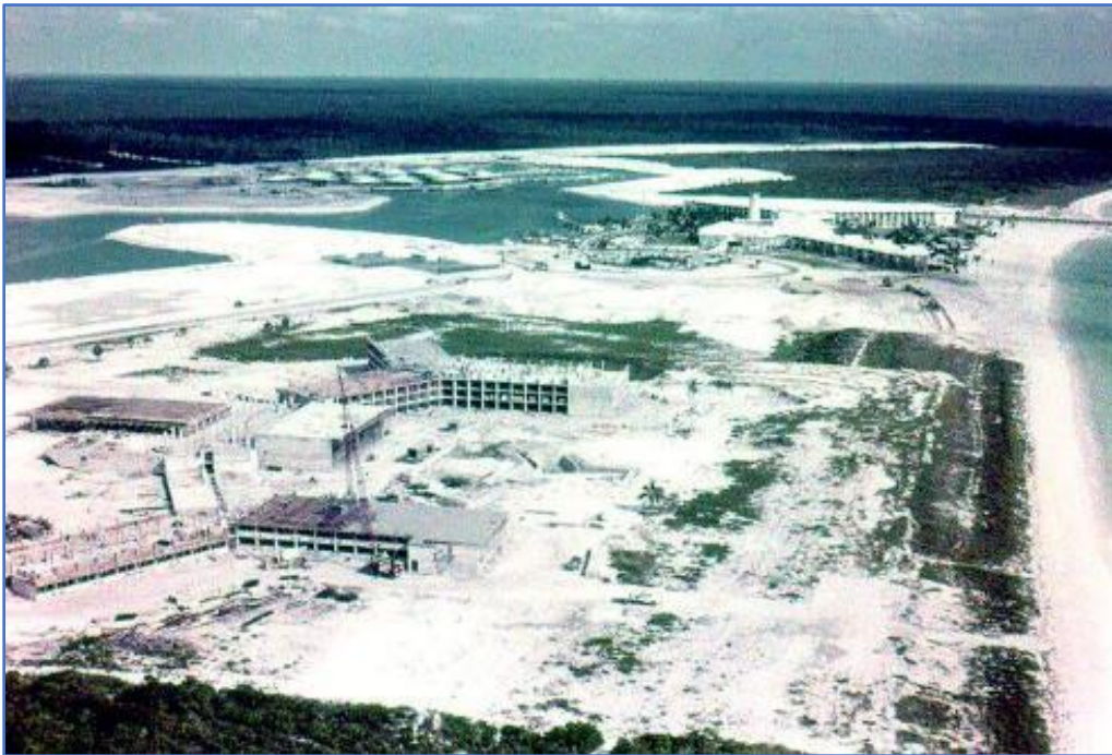
Figure 11-2. Holiday Inn Under Construction and Lucayan Beach Hotel in Background.
