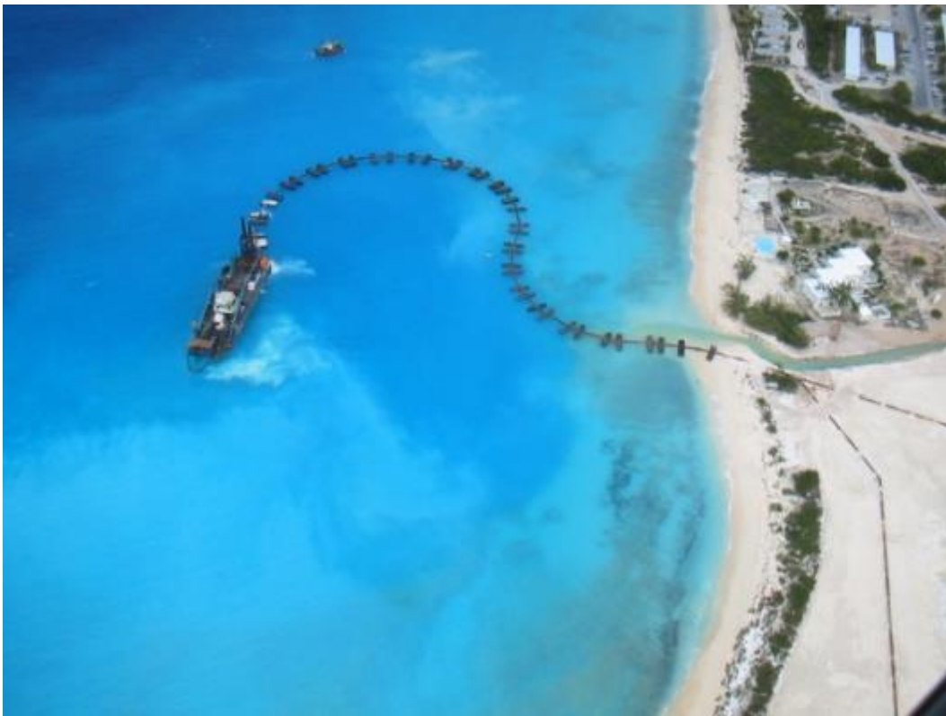
Photo 6.1. Representative photo of hydraulic dredging (Grand Turk Cruise Facility construction)
