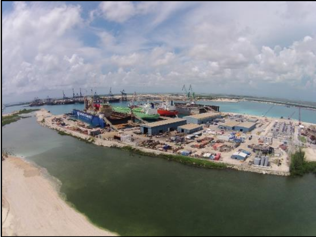
Figure 2-8. Aerial Photograph of the Grand Bahama Shipyard (September 2014) Source: Envirollogic International
